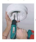
Step 1: Secure Housing to Mounting Surface
