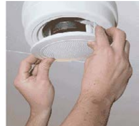
Step 3: Fit Speaker to Housing
