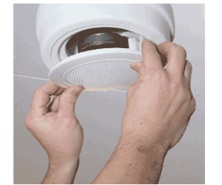
Step 3: Fit Speaker to Housing
