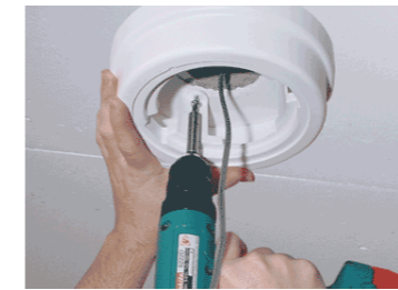
Step 1: Secure Housing to Mounting Surface
