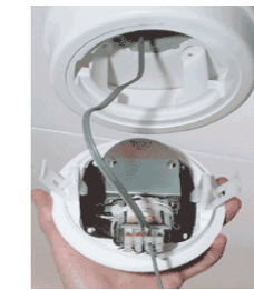
Step 2: Terminate Cable
