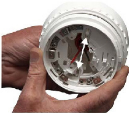
Snapping the detector base to the CTA Back Box
