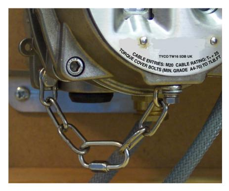
Fig. 32 Safety Chain Connection
