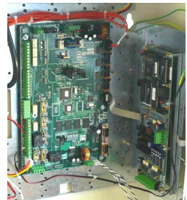
Figure 27 I-HUB Mounted on right side Flange
