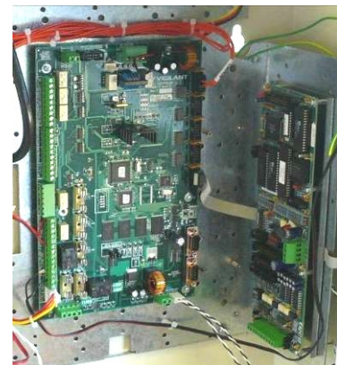
Figure 16.4 – I-HUB Mounted on right side Flange
