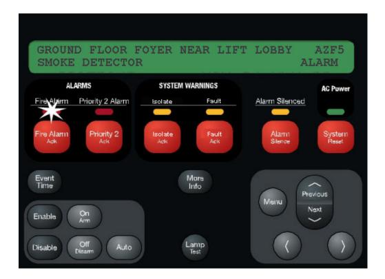
Figure 2-1. Alphanumeric Display Showing Typical Alarm
