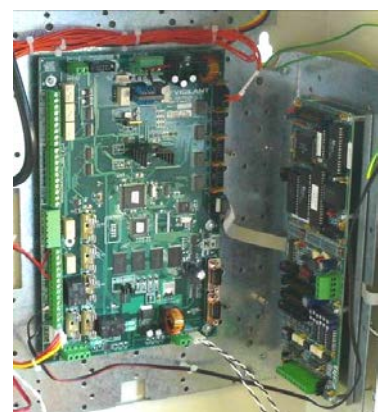
Figure 11-25 I-HUB Mounted on right side Flange
