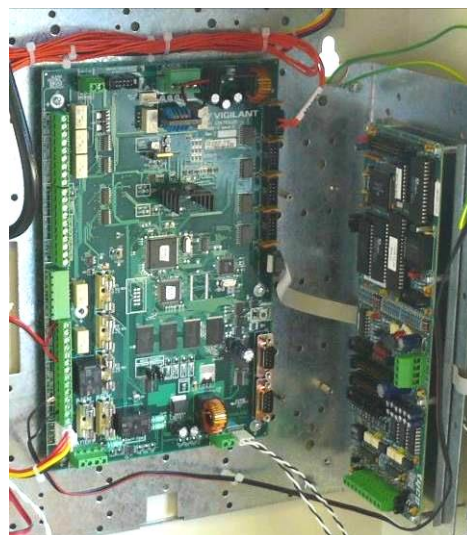
Figure 14.3 – I-HUB Mounted on 15U Gearplate RHS Flange
