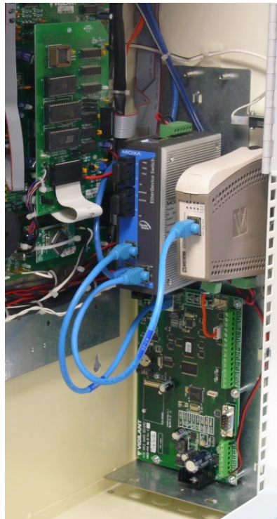
Figure 4-4 – FP1013 Bracket in 15U Cabinet Mounting PIB, Switch, Ethernet Extender
