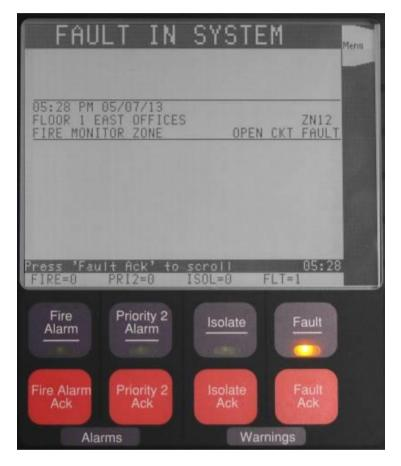
Figure 3-1. Operator Interface Showing Fault Condition
