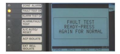
Figure 5-2. Ready for Zone Fault Test
