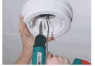
Step 1: Secure Housing to Mounting Surface
