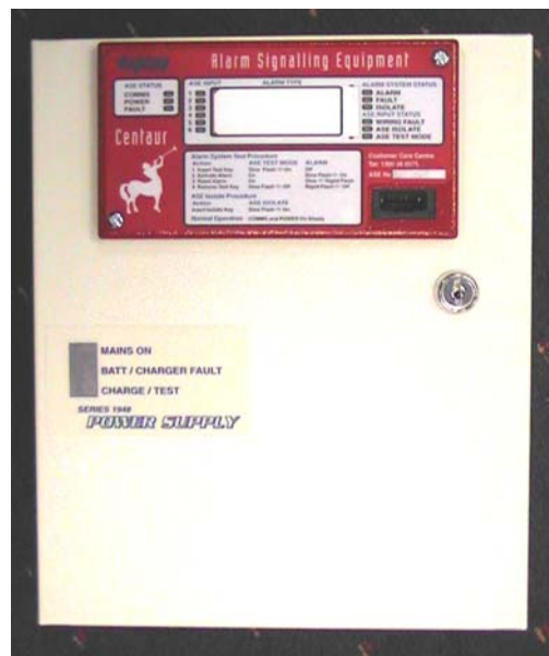
Figure 9 – ASE with power supply unit
