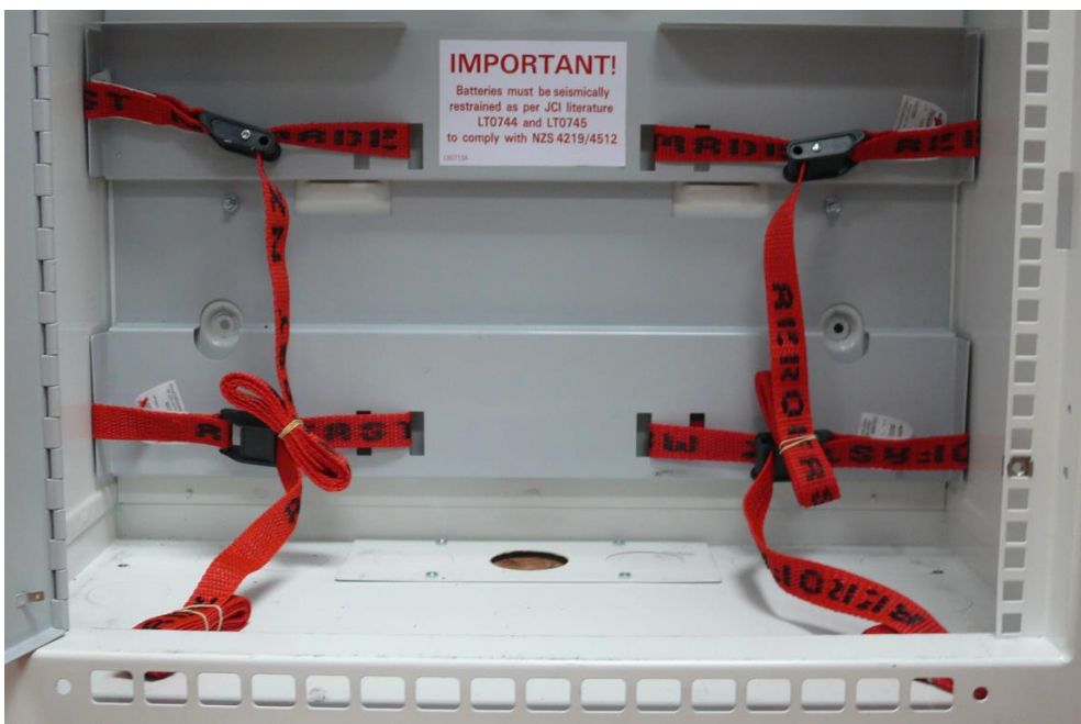
Figure 4 – Mounted Battery Restraining Bracket
