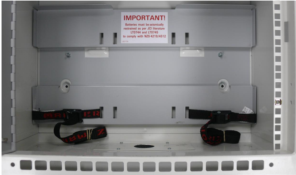
Figure 1 – Mounted Battery Restraining Bracket
